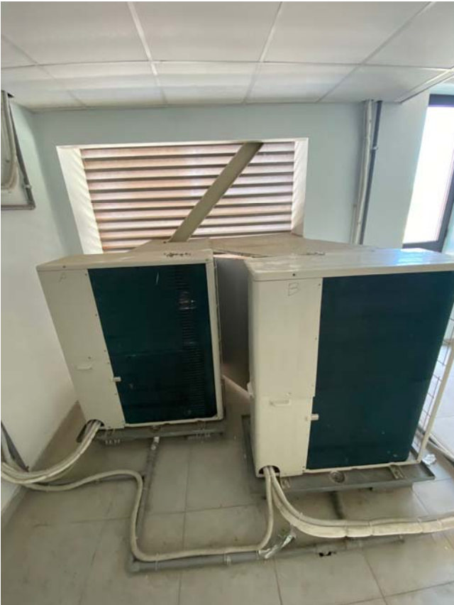
Unità esterne: TOSHIBA modello MCY-MHP0604HS8-E (18,00 Kw) - TOSHIBA modello MCY-MHP0504HS8-E (16,00 Kw)
